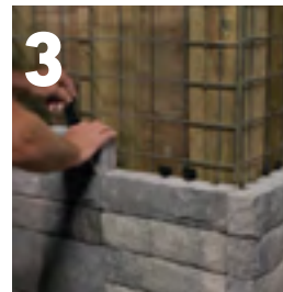
3 Attach Tandem Veneer with Connector
