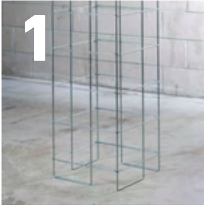
1 Start with Column Grid
